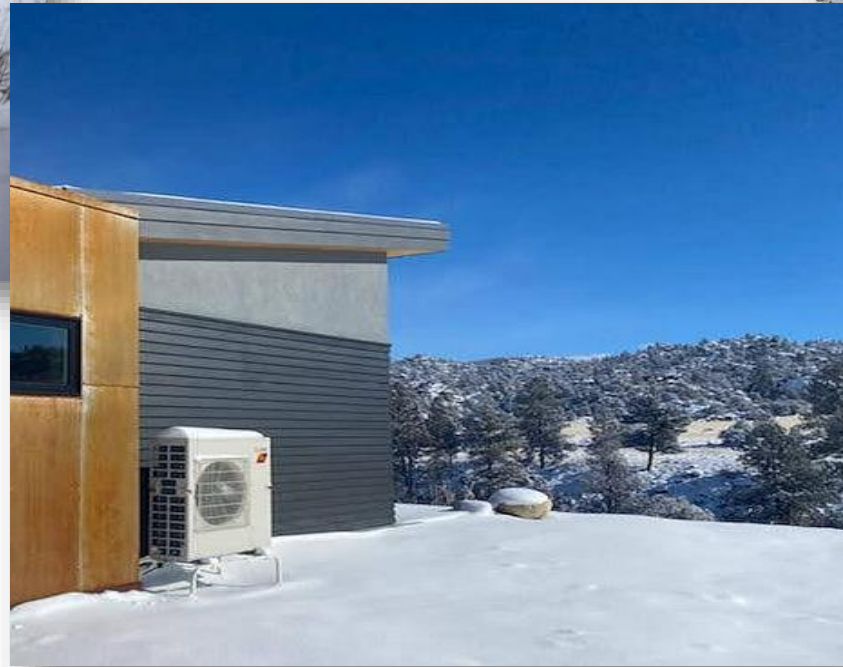
7,600 ft elevation -22F and “very comfortable” operating beyond specification
