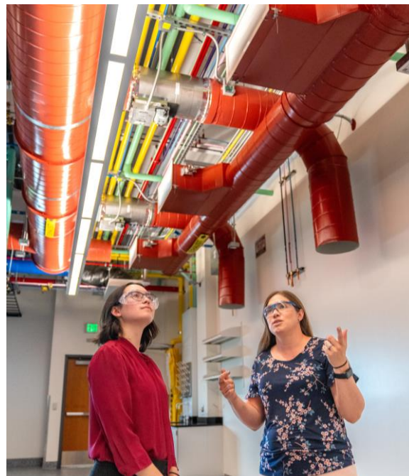
Photo by Werner Slocum / NREL
